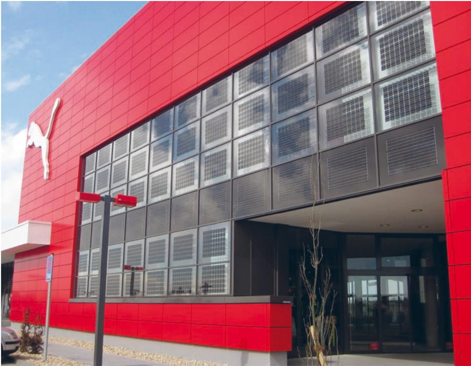
Striking Solar Power: Photovoltaic cells integrated into the facade of the PUMA Store at the new PUMA Vision Headquarters in Herzogenaurach, Germany
